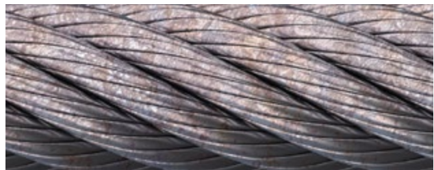
Fig.: Slight corrosion, 0% - 20% severity
