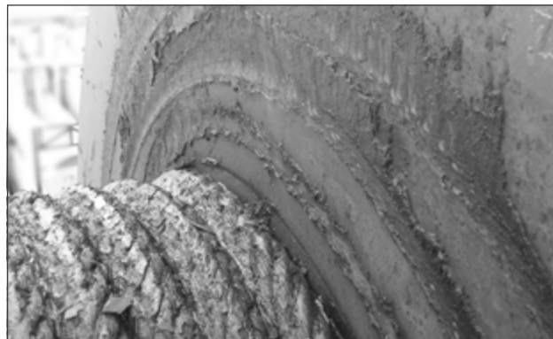
Fig.: Wear on a drum flange
